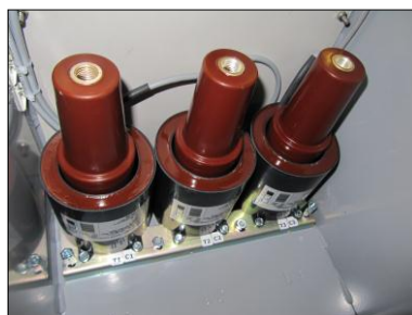
Cones type C Circuit-breaker 500 A incl. current transformers
