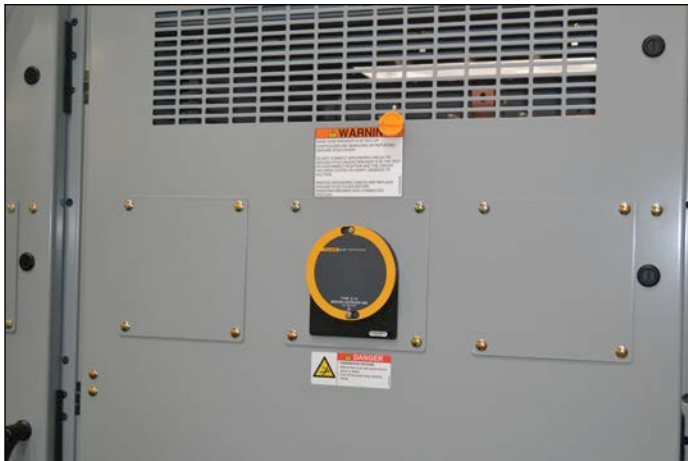
Figure 5.4-6. Typical Install for IR Window on Rear Door
