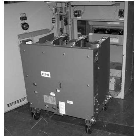
VCP-W Direct Roll-in Breaker with Fixed Wheels
