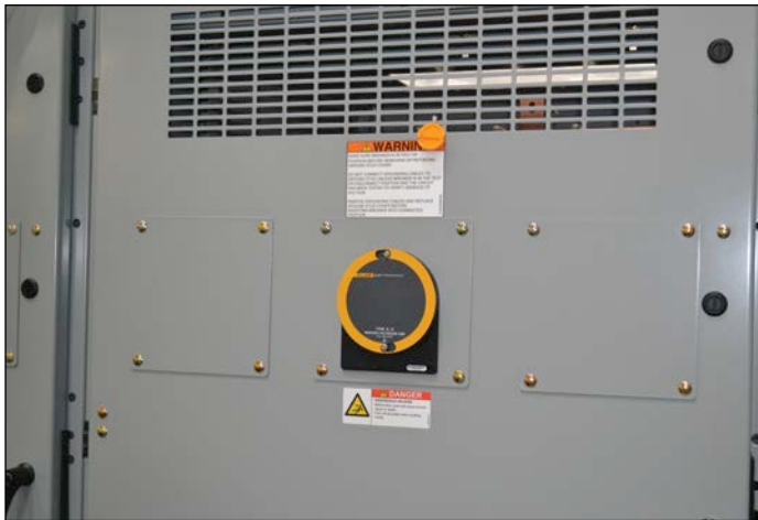
Figure 5.1-9. Typical Install for IR Window on Rear Door
